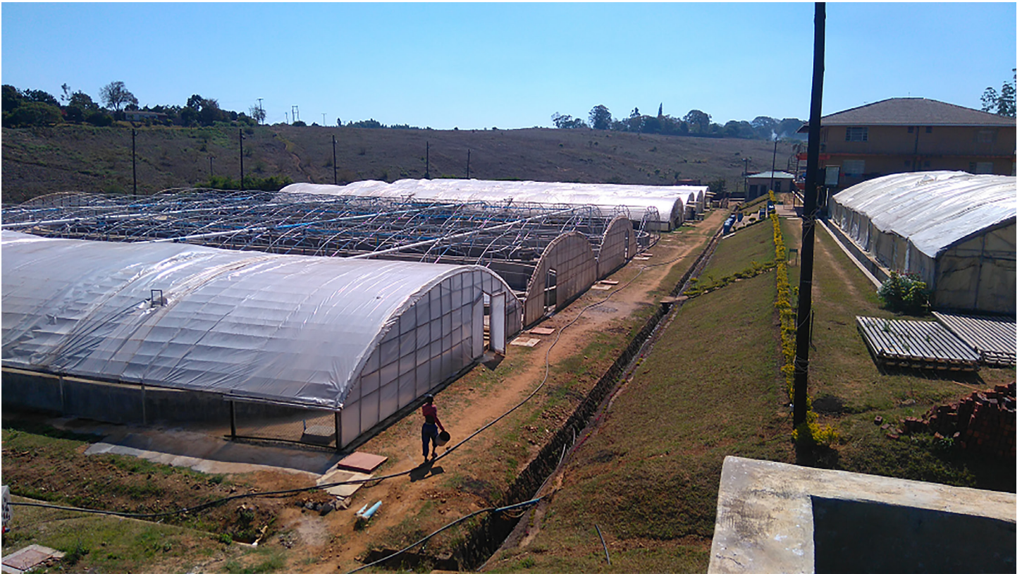
Figure 3. A battery of eight 766-m 3 multi-cohort sequential SAFF-BFT grow-out tanks at Chambo Fisheries near Blantyre, Malawi.
